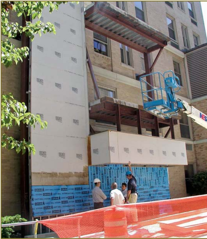
Figure 2 – Construction of an on-site, stand-alone mock-up.
