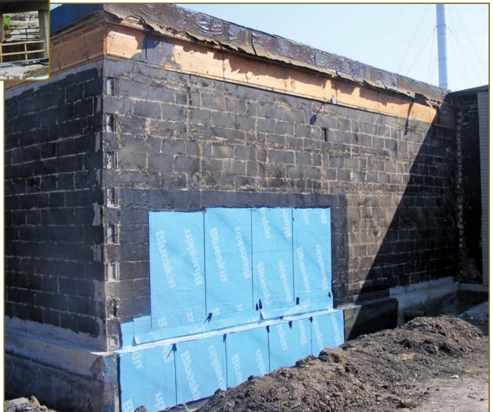
Figure 4 – Mini mock-up of air barrier installation.
