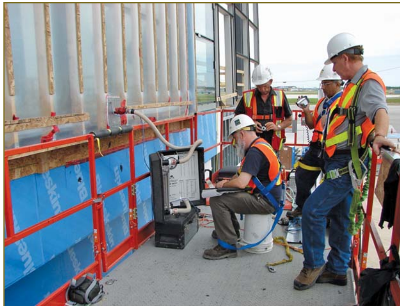
Figure 7 – On-site air infiltration testing of window-wall mock-up.
