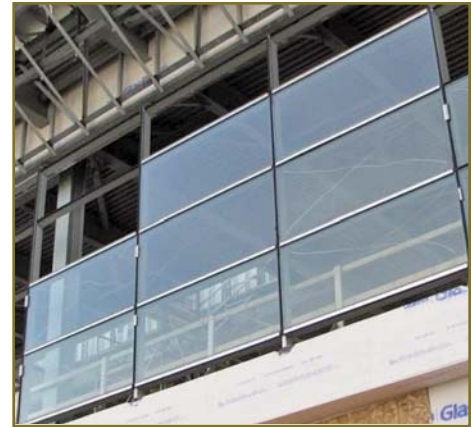
Figure 5 – Aesthetic mock-up to view appearance of glazing.
