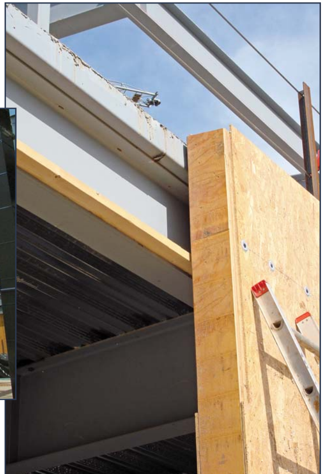
Figures 3A and 3B – Dimensional lumber nailers were attached to the structural steel frame of this Cherokee Nation school in North Carolina. The SIPs were attached to the nailer using SIP screws through the thickness of the panel.
