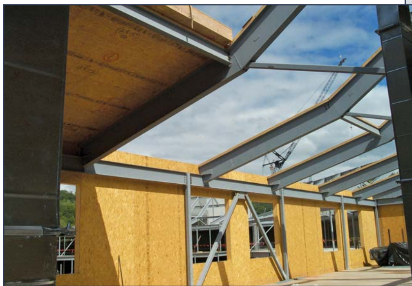
Figures 3A and 3B – Dimensional lumber nailers were attached to the structural steel frame of this Cherokee Nation school in North Carolina. The SIPs were attached to the nailer using SIP screws through the thickness of the panel.
