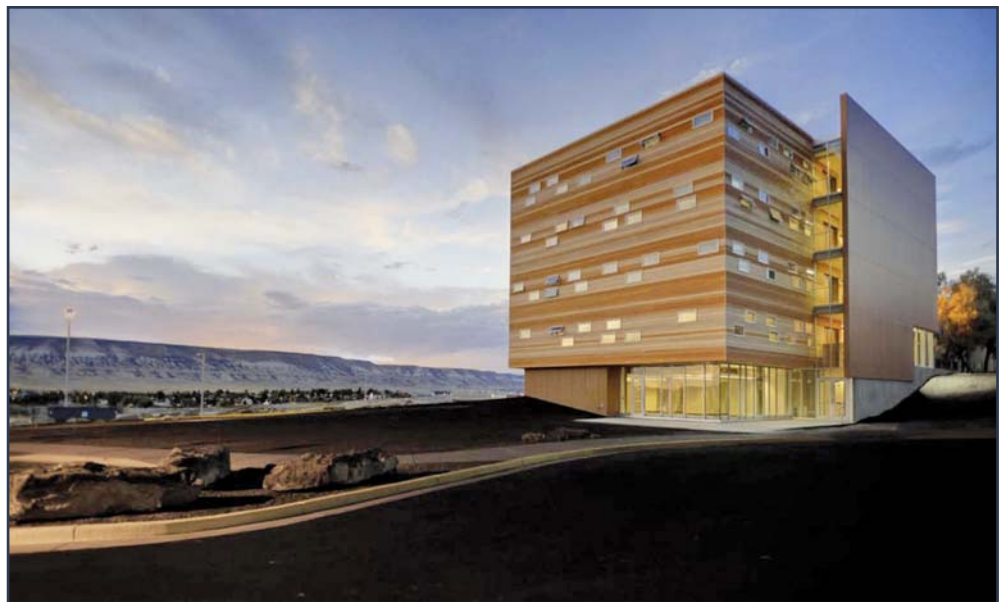
Figure 2 – Wind River Hall student housing at Western Wyoming Community College is a four-story self-supporting SIP building. Kamerman Construction estimated that SIPs shaved two to three weeks from the construction schedule.
