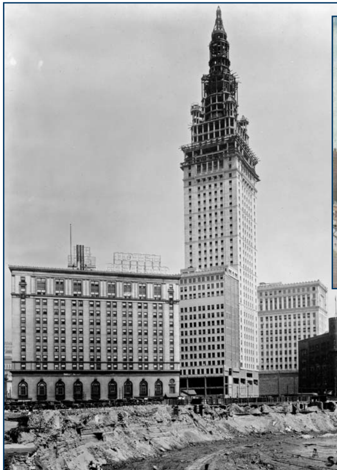
Figure 1 – Skeleton-frame building under construction (image from www.skyscrapercity.com ).
