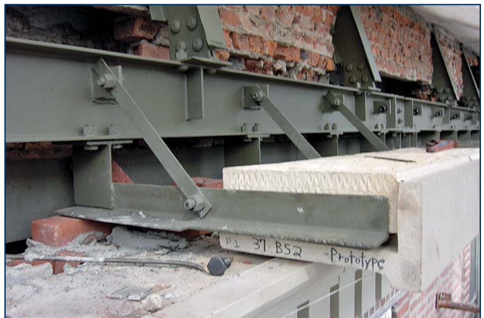
Figure 11 – Coating of existing steel support with corrosion-inhibiting system.
