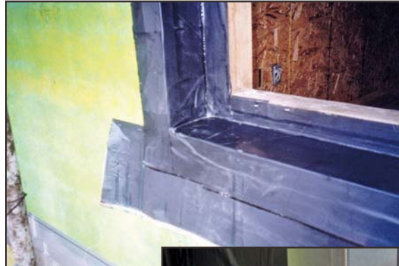
1: Type III – SAF pan – concealed for nail-fin window in recessed metal siding opening.
