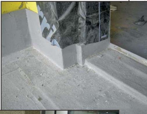
7: Type I – GSM pan – Concealed, for block-frame window in recessed stucco opening. Type III SAF sill pan under the metal pan.
