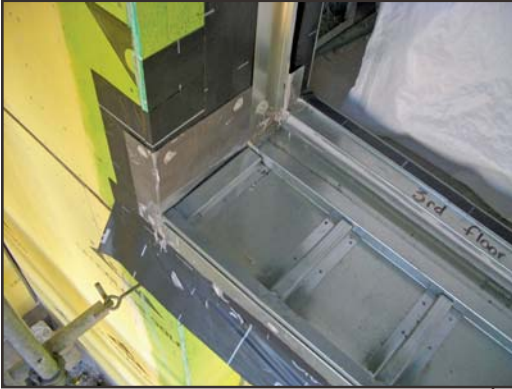
7: Type I – GSM pan – Concealed, for block-frame window in recessed stucco opening. Type III SAF sill pan under the metal pan.
