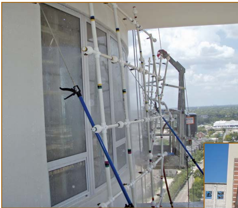
Photo 4 – A water spray is constructed to test windows on a slight radius on a high-rise building in Houston, TX. Part of the window assembly extends past the edge of the balcony, so swing-stage equipment was utilized to support portions of the water-spray rack during the testing.
