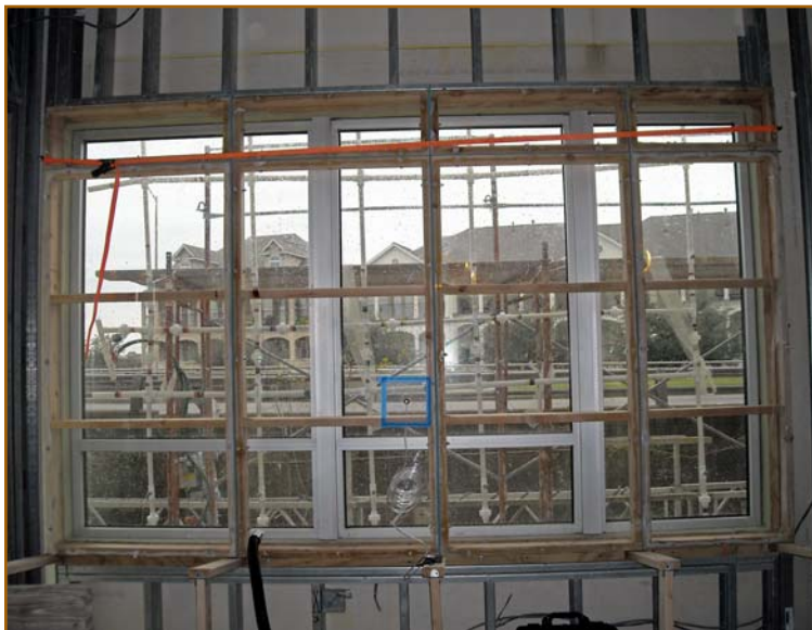
Photo 1 – An interior-mounted pressure chamber on a large, triple-mulled window assembly on a project in Houston, TX.
