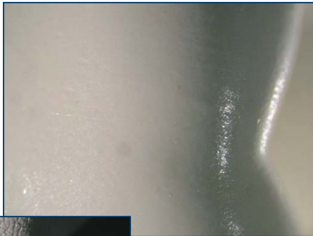
Photo 6 – PVC membrane #3 (initial).
