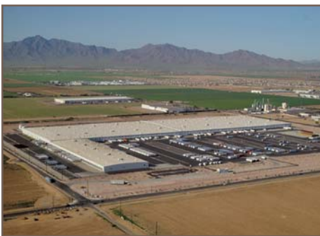
Figure 1 – Overview of roof recently instrumented to gather information about wind uplift pressures and roof system fastener loads associated with actual wind gust events (source: Google Earth Pro).
