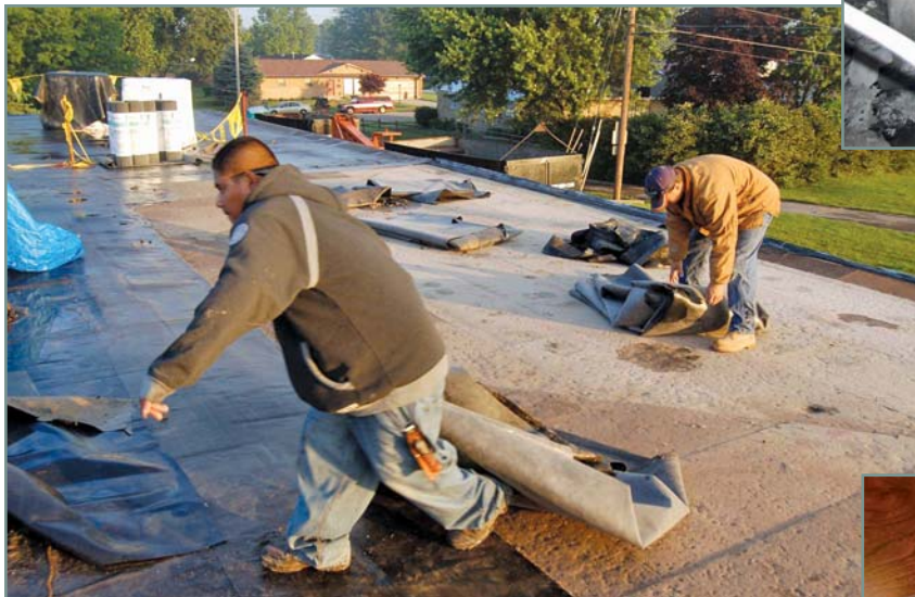
Photos 1, 2, and 3 – EPDM is removed from a ballasted system (above, left). Afterward, it is taken to the grinder (top right), and the final product results (bottom right). (Photos courtesy of ERA.)
