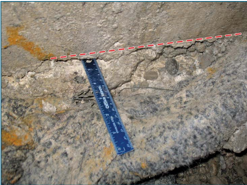
Figure 9 – Channel-like cavity in footing between smooth side (above dotted line) and bulge.
