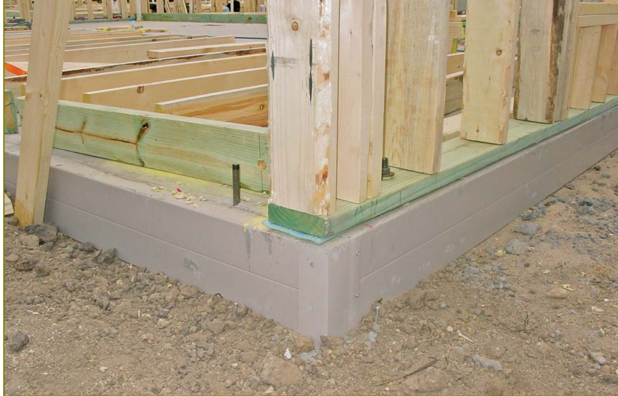
Figure 2 – EnergyEdge® remains in place as part of the foundation, leaving a finished and insulated slab edge with an R-10 thermal resistance value, meeting International Energy Conservation Code (IECC) requirements.
