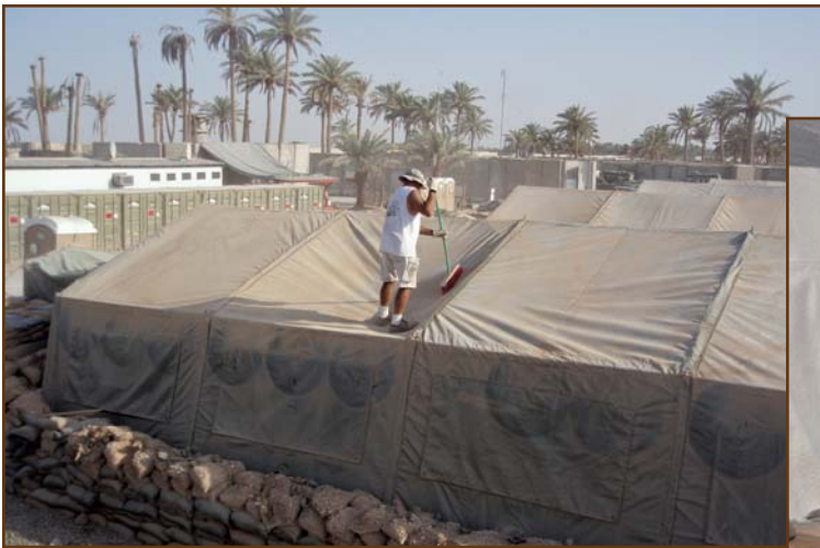
Tent cleaning (left) prior to foam application.
