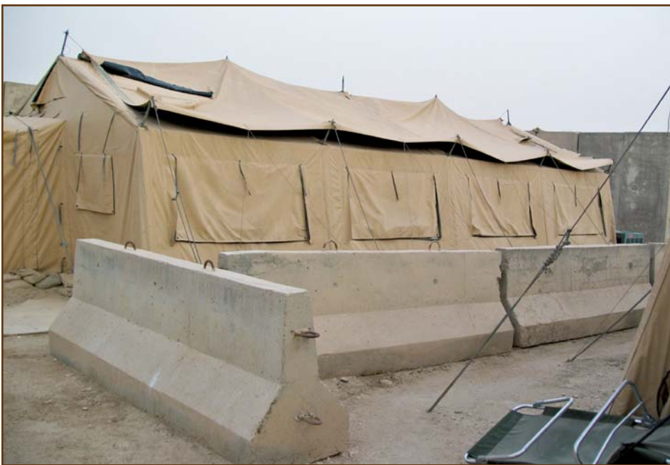
Typical tent before spray foam application.
