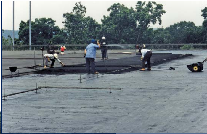
Figures 5 and 6 — Ordinarily installed over a structural concrete deck, All-Weather Crete is more appropriately termed a “substrate” for the eventual roof covering. Here, the ball field (occupied below) at Georgetown University receives what resembles a roadway pavement topping.
