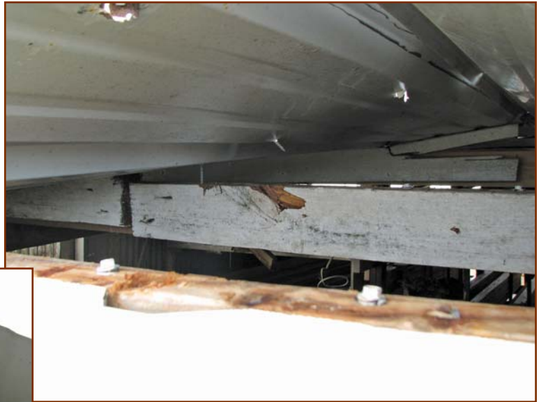
Figures 7 (right) and 8 (below) – Fasteners pulled through the new metal skin where there was no ccSPF to help secure the panels to the wood trusses.
