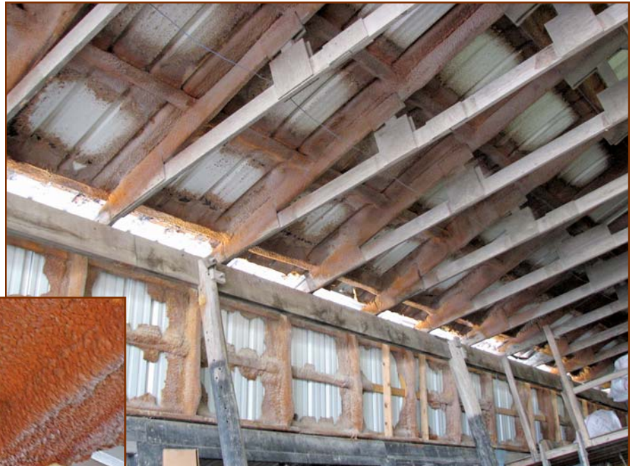
Figure 5 – Old metal secured with ccSPF.
