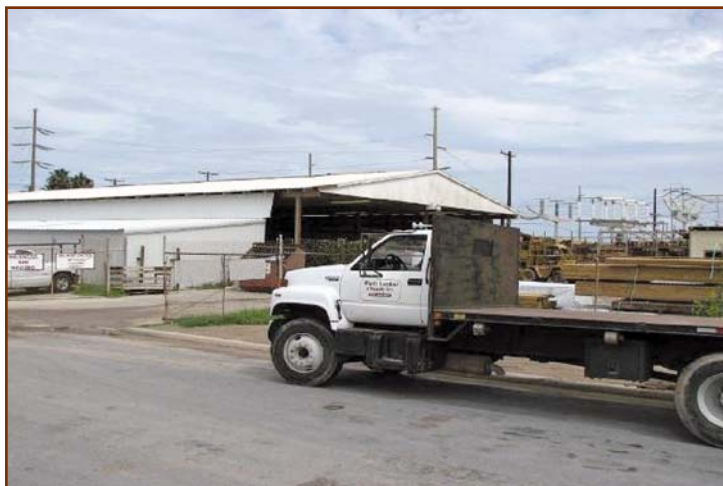
Figure 2 – The author installed the old metal roof on this building in 1980. A new metal roof was installed in 2008 on the right side of the building.
