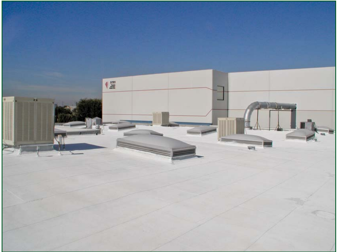
While it may make more sense economically to replace an older roof near the end of its life cycle, a newer roof still in good shape can be economically transformed into a cool roof that will rival the effectiveness of a new, manufactured cool roof.
