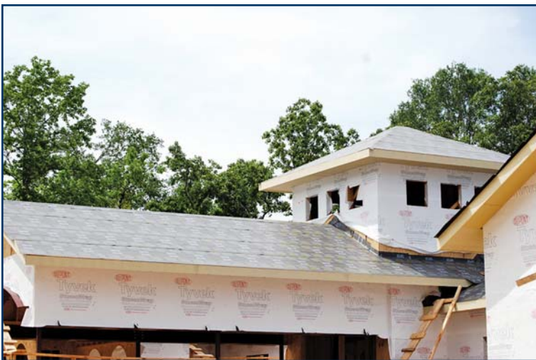
Figure 5 — LeakBarrier PS200MU Ice and Water Armor is a self-adhesive, glass fiber-reinforced, modified bituminous underlayment especially for metal roofing. It helps protect a building's deck or internal structure against leaks caused by ice and water damming and wind-driven rain.
