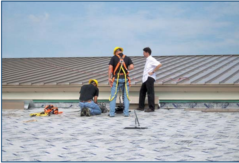
Figure 4 — Metal panels are being installed over PS200HT self-adhering underlayment, which provides a smooth surface and resistance to high temperatures.
