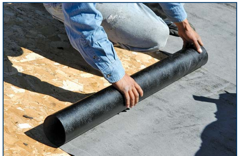
Figure 1 — EasyLay® asphalt-saturated high performance polyester handles the same as traditional felt, yet offers the advantages of a synthetic felt.
