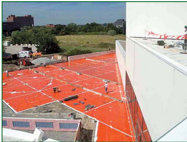
Photo 9 – Thermoplastic waterproofing membrane/grid system.
