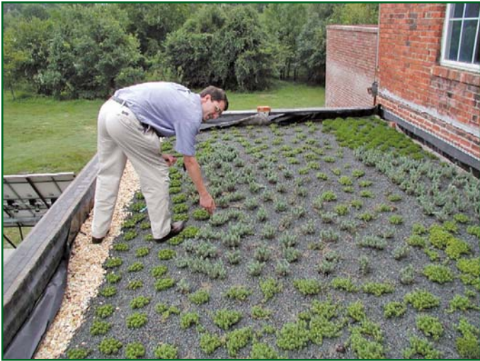
Photo 4 – Installation of media and planting.
