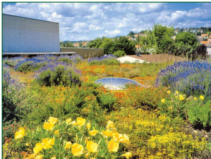
Photo 5 – Extensive green roof assembly.
