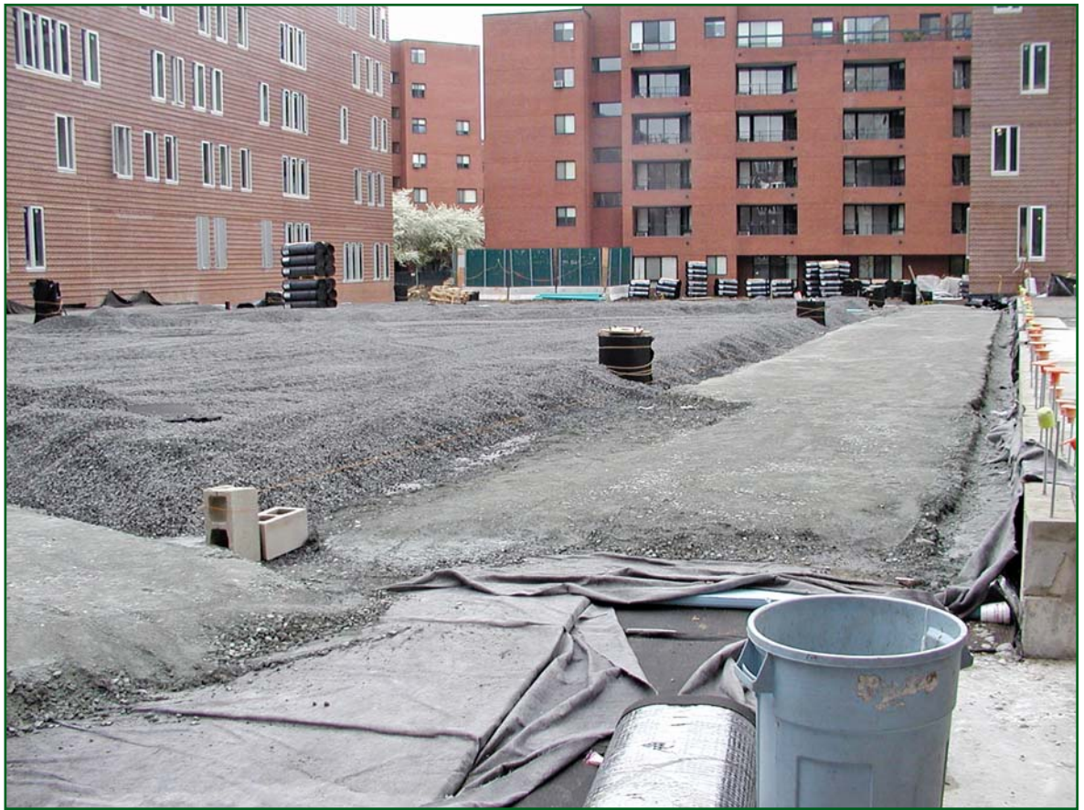
Photo 8 – Various media layers being installed.
