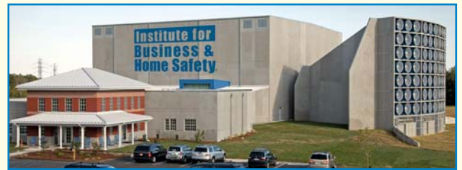
The new IBHS multirisk building science center opened in Chester County, SC.
