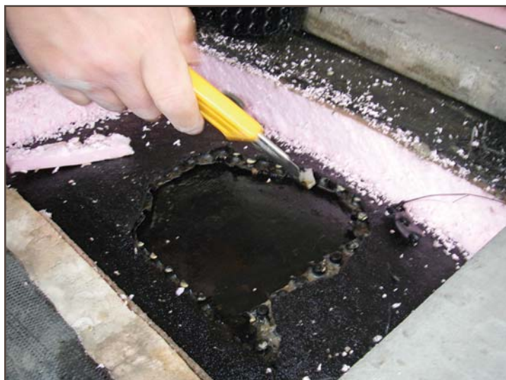
Figures 11 and 12 – Cutting of membrane blister and expulsion of water during extraction process.
