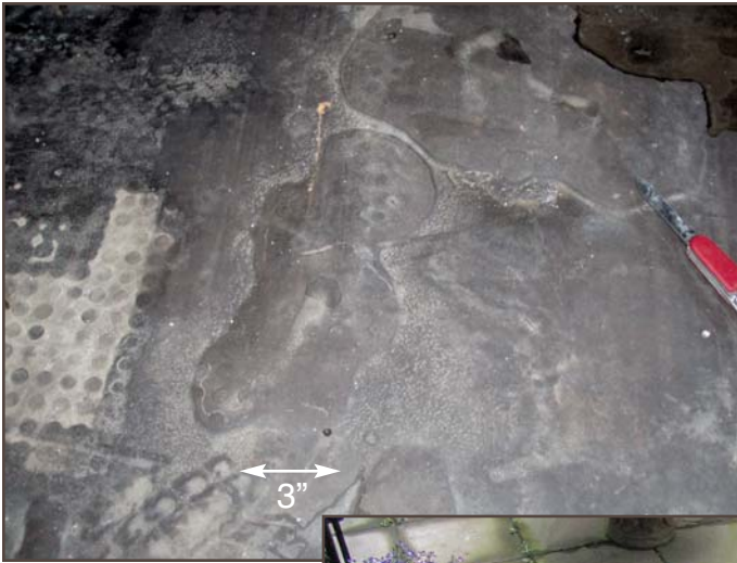
Figures 1 and 2 – Typical blistered roof membranes. Blisters range from penny sized to areas several square feet in a 5- to 10-year-old membrane.
