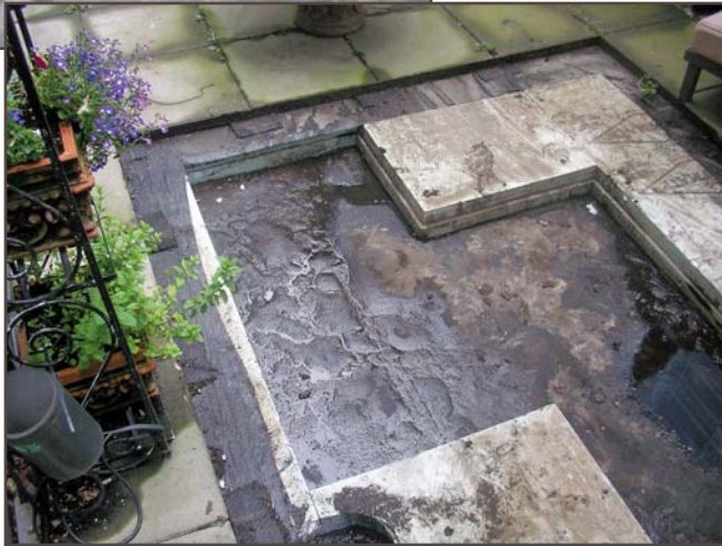
Figures 1 and 2 – Typical blistered roof membranes. Blisters range from penny sized to areas several square feet in a 5- to 10-year-old membrane.
