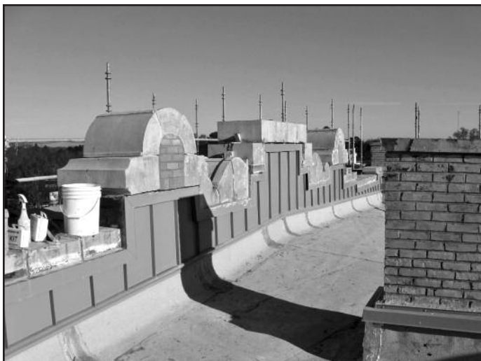
Photo 15 – Installed rainscreen at back side of parapet wall.
