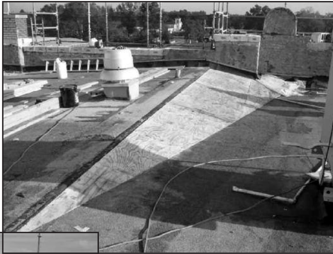
Photo 3 – Steep-slope cricket at existing transition in roof slope.
