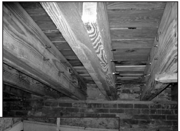
Photo 7 – View of sistered rafters from beneath after deck reinstallation. Note masonry knee wall.
