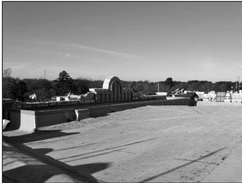
Photo 20 – Completed roof system.
