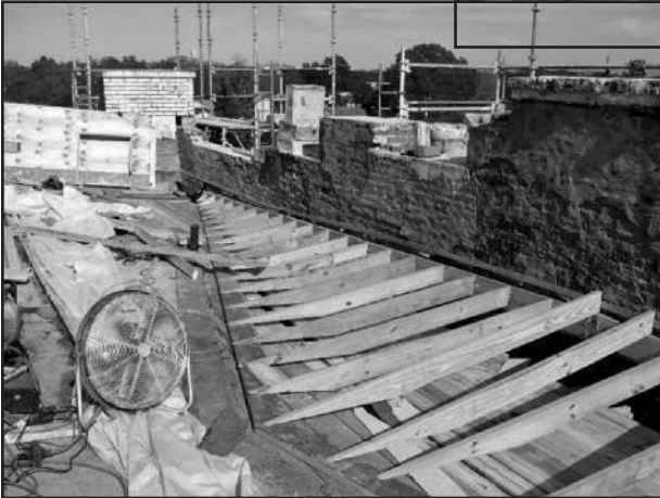
Photo 4 – Steep-slope cricket at parapet wall.
