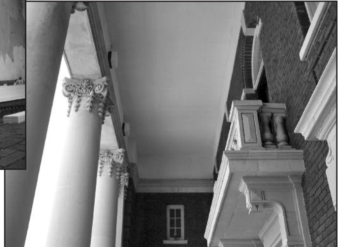
Photo 9 – New portico ceiling slab.
