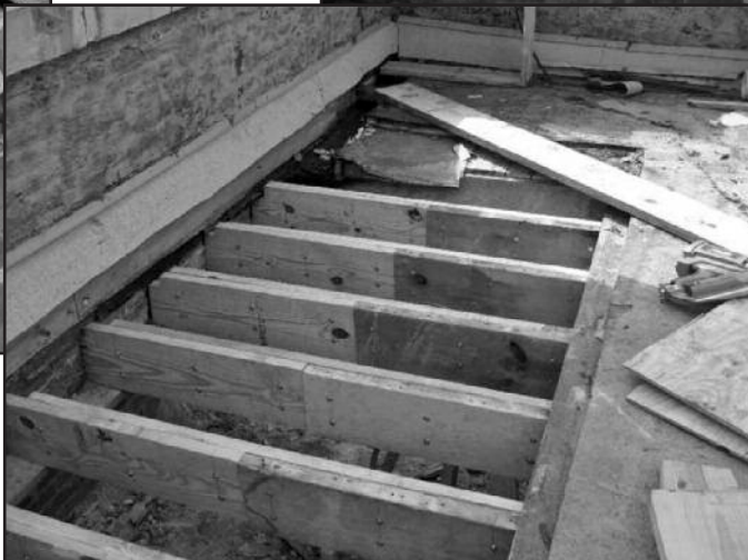
Photo 6 – View of sistered rafters from above prior to deck reinstallation.
