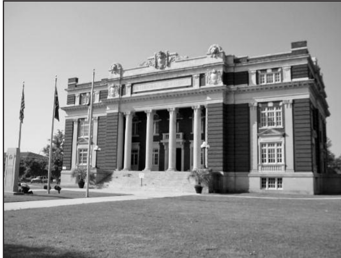
Photo 1 – Overview of building façade.
