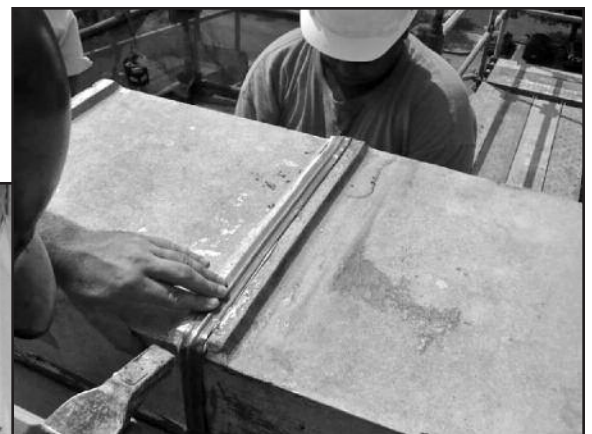
Photo 12 – Installation of lead cap at terra-cotta sealant joints.
