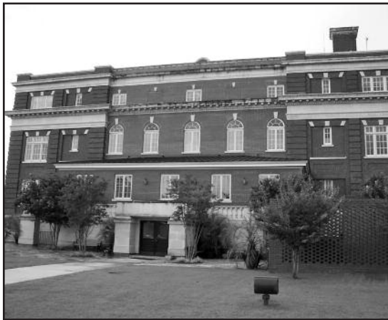
Photo 13 – Rear elevation of addition before restoration of parapet.
