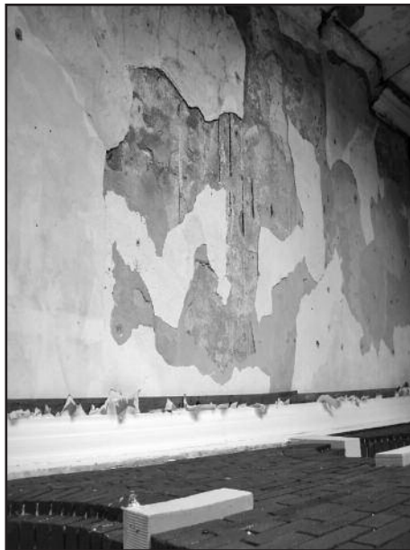
Photo 8 – Underside of portico ceiling at start of project.
