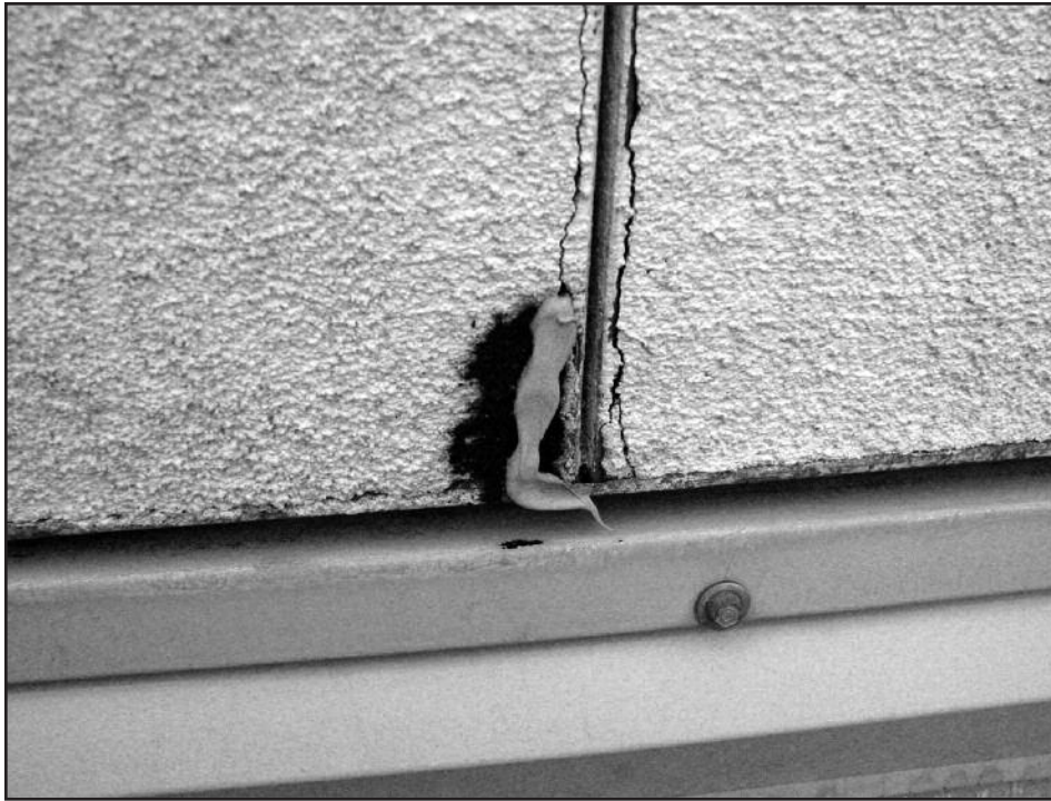
Photo 6 – Does this condition require further investigation?
