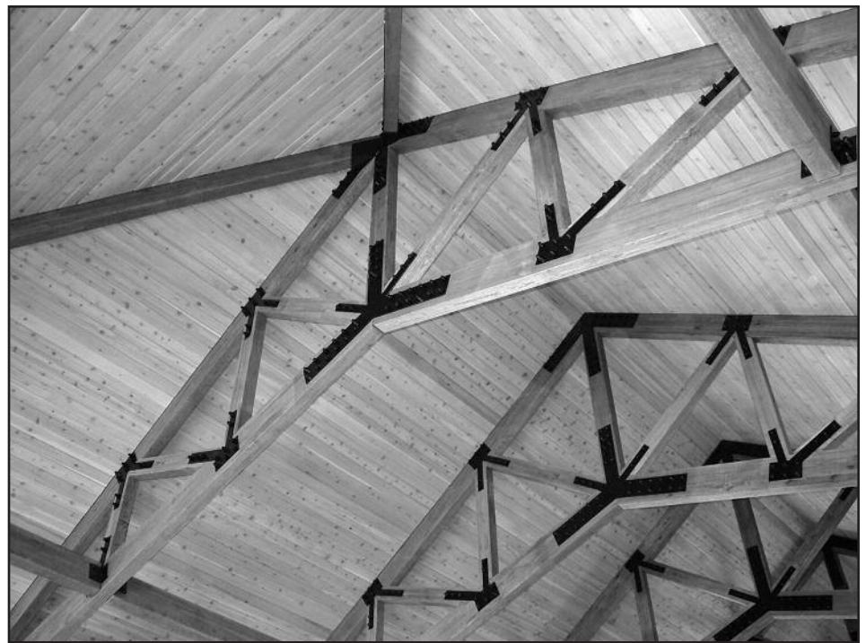
Figure 4 – View of the pool roof heavy-timber trusses and cedar-ceiling finish.
