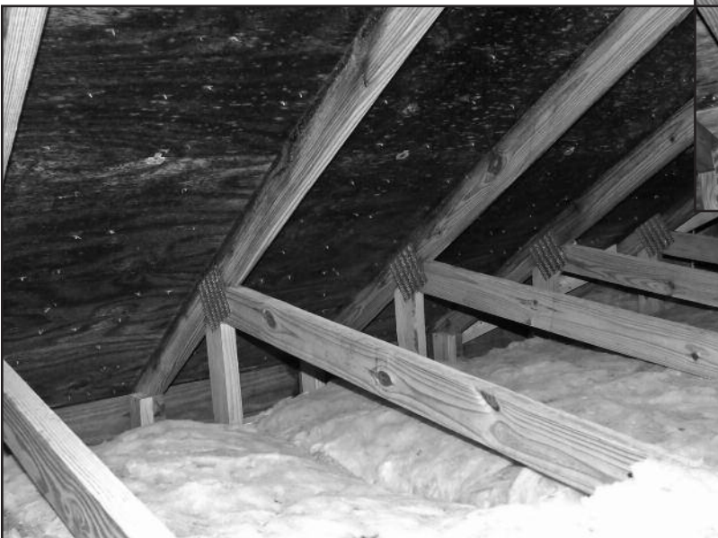
Figure 11 – Biological growth on sheathing in attic space above equipment room prior to occupancy.
