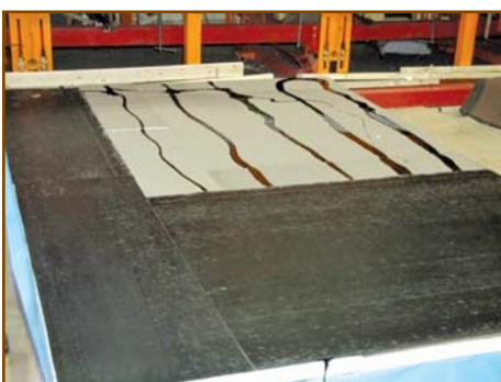
COVER BOARD INSTALLATION
