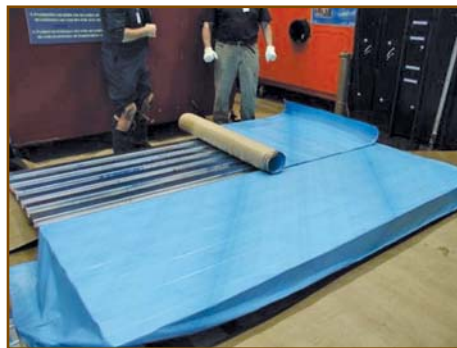
VAPOR BARRIER INSTALLATION
