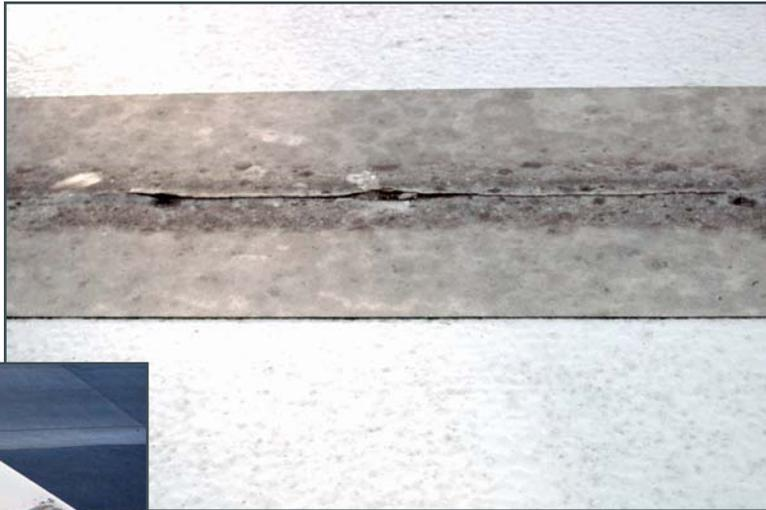
Figure 5 — Adhesive failure
