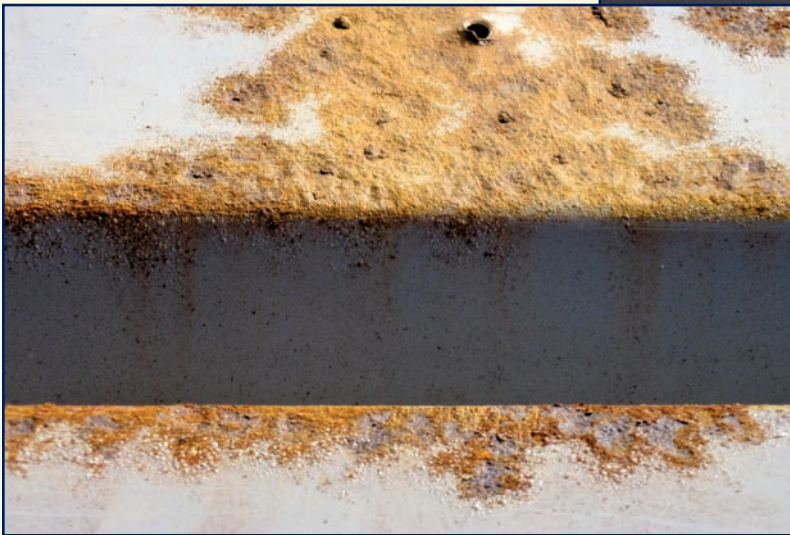
Photo 7 — A close-up of Photo 6 shows pitting and scale are developing. This was a former plate-and-screw location; the condition appears to accelerate at these locations.
