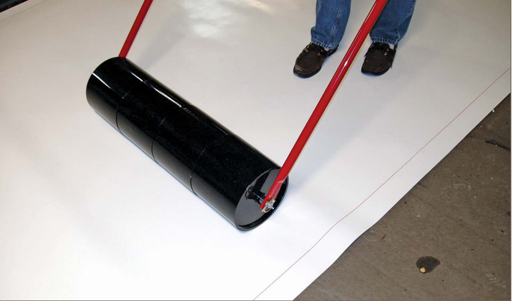
Photo 5 — Rolling membrane with weighted roller
