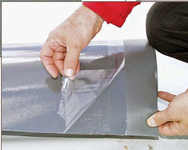
Photo 3 — Removal of backing from membrane
