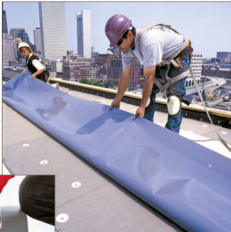
Photo 4 — Folding down membrane
