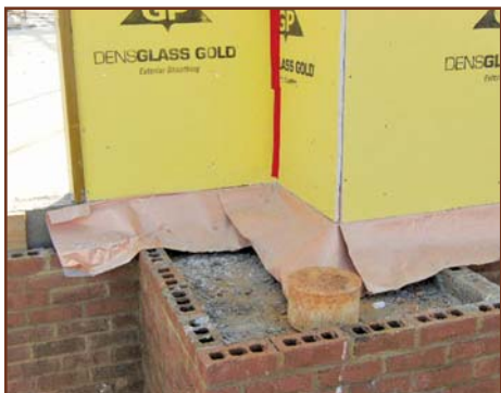
Figure 12 – Flashing properly located behind sheathing and joints overlapped but not yet sealed.
