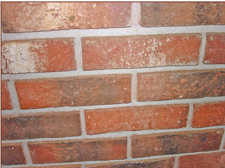
Figure 7C – Tooled raked joint.
