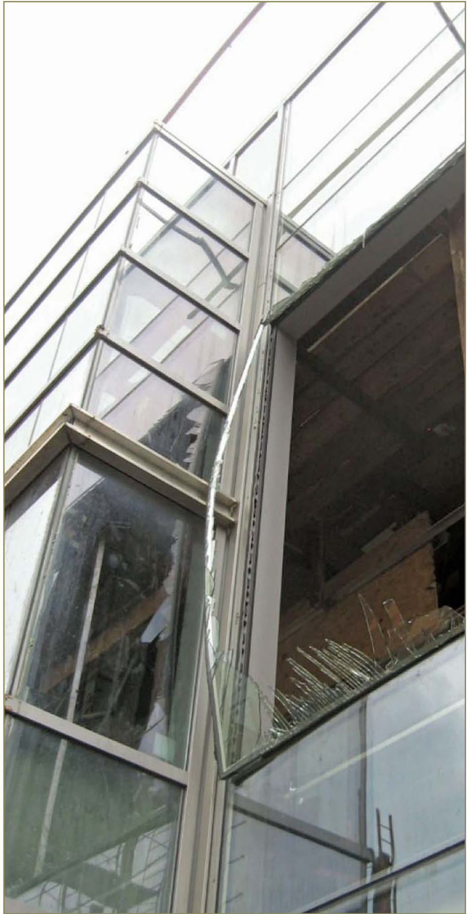
Photo 11 - Curtain wall after 150% design load test.
