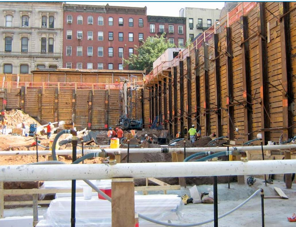
*Photo 1 – Soil retention system to receive blindside waterproofing at zero lot line foundation.*
