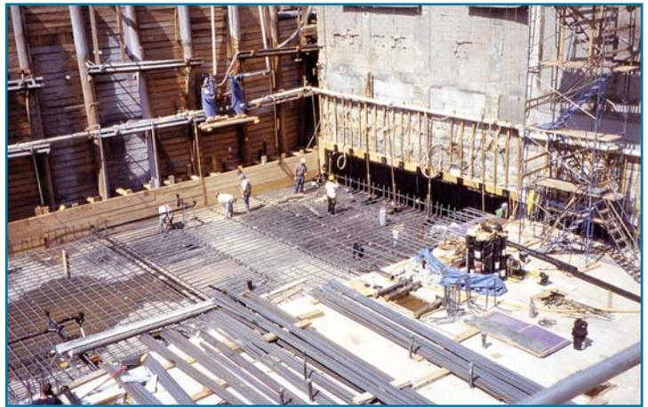
Photo 2 – Bituminous membrane installed under pressure slab and boarded-out lagging.
