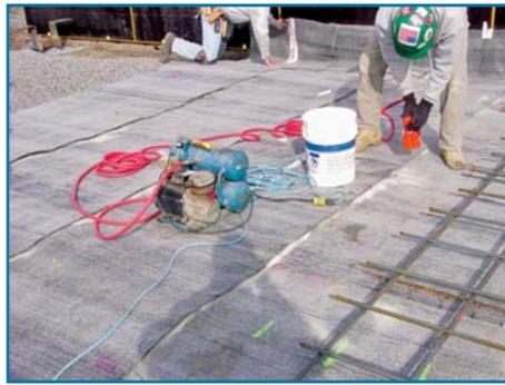
*Photo 5 – Bentonite membrane under pressure slab.*
