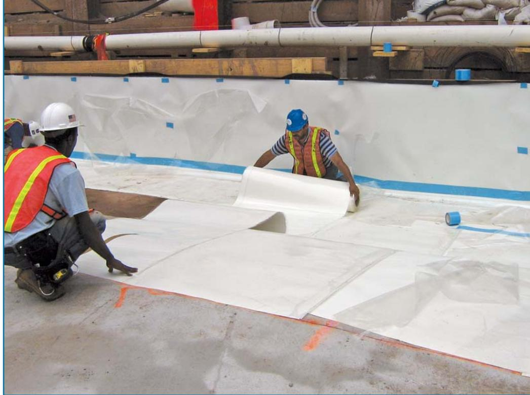
*Photo 3 – HDPE sheet membrane on mud slab and lagging.*
