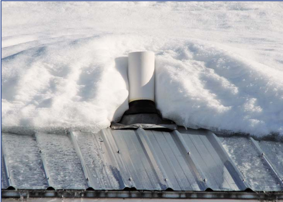
Figure 5 – Standard 3-in plumbing vent prevents snow from sliding off a metal roof.
