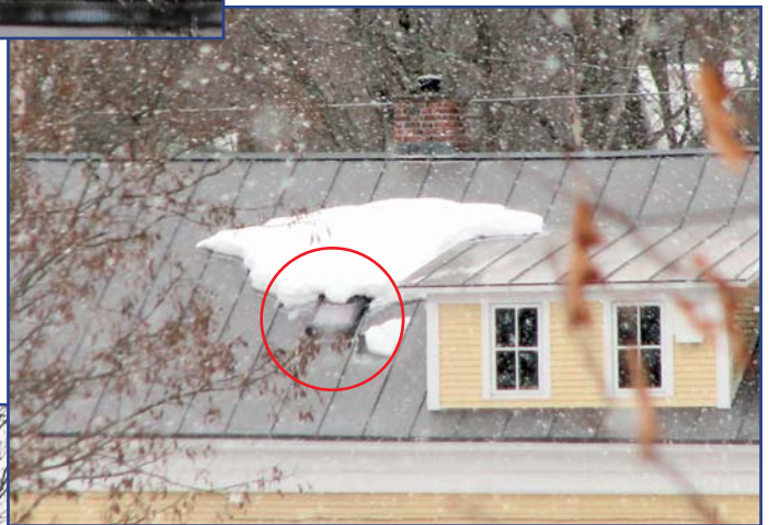
Figure 6 – Small skylight holds back an inordinate amount of snow relative to its size.
