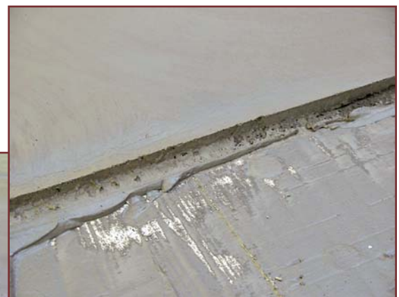
Figure 8 – End-of-the-day cold joint for following day tie-in.
