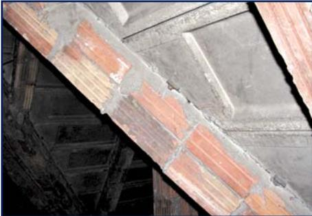
(Figure 2). Most multistory buildings of decades past having this type of roof deck might also have this arrangement as the floor-to-floor construction.
