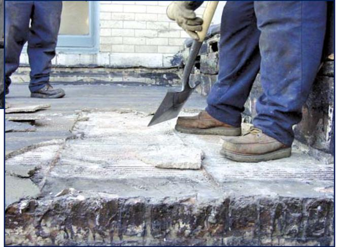
Figure 8 – Delamination and spalling of mortar topping course.
