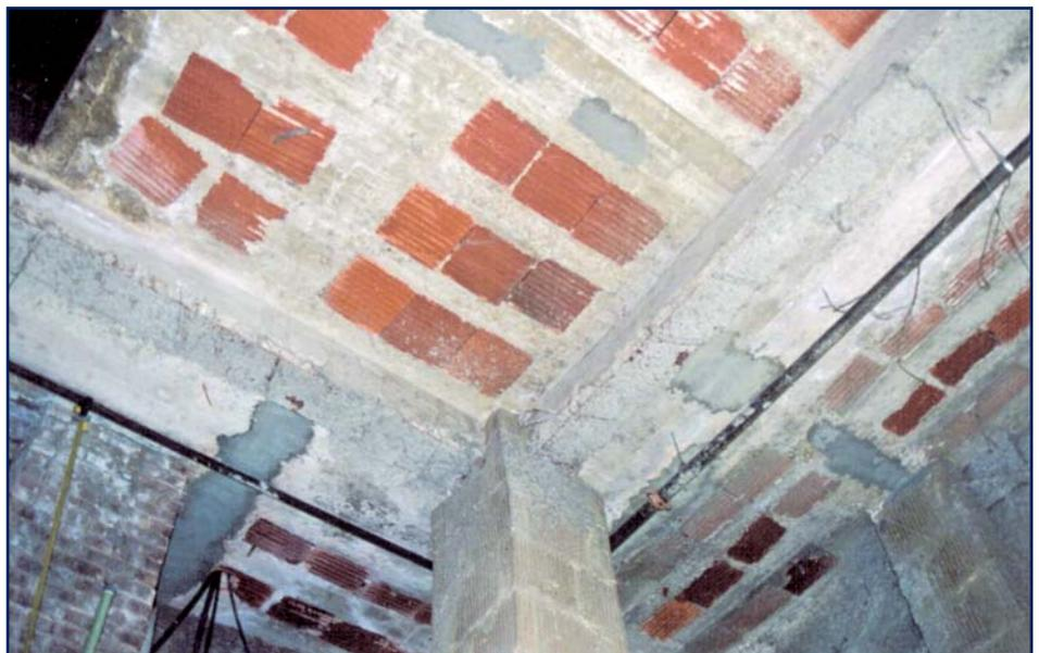
Figure 4 – The common arrangement of tiles nested onto sloped steel framing. Additional mortar would be struck into joints from the roof (top) side.
