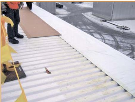
**Photo 5 – FRP roof decks are a suitable substrate for either single-ply or built-up roofing.**
