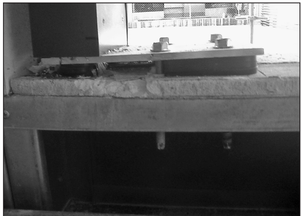
Figure 11 – Curtain wall mullion F bracket installed on gypsum sheathing at sill.
