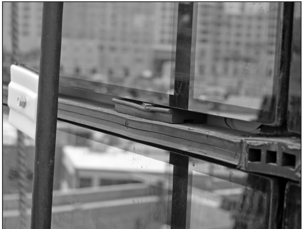
Figure 13 – Placement of shim above setting block.
