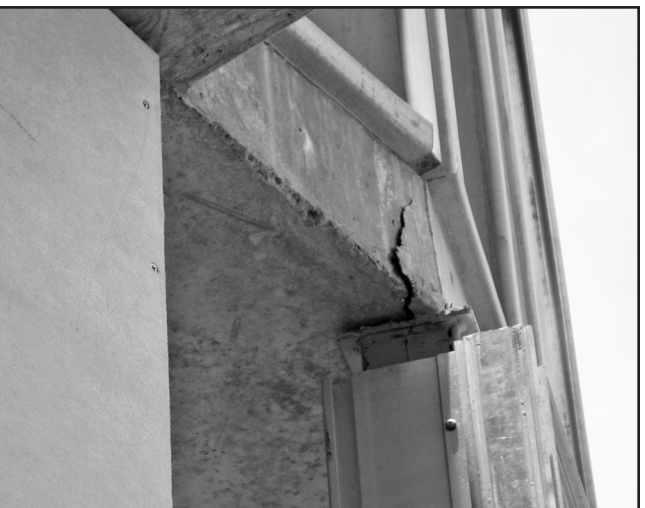
Figure 2 - Concrete distress at mullion-head connection due to lack of adequate edge distance.
