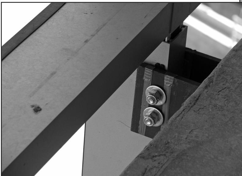
Figure 2 - Concrete distress at mullion-head connection due to lack of adequate edge distance.
