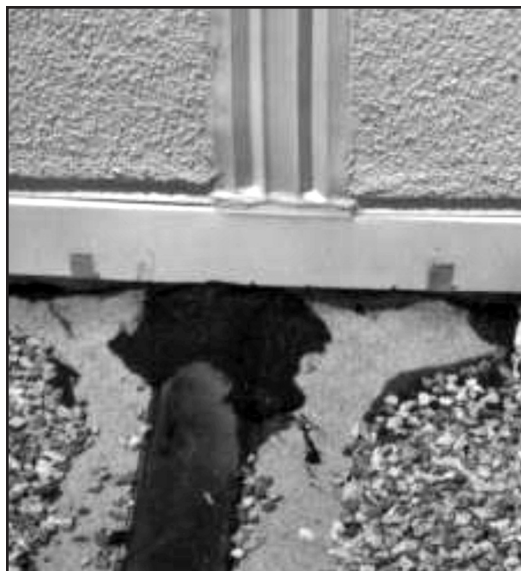
Photo 4 – Closures never meet and flashing is not split.
