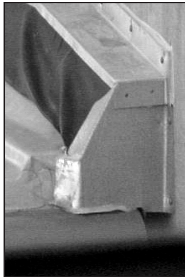
Photos 7 and 8 – These two photos show the same basic condition. Both use bellows for the flexible closure. Photo 7 is capped with a metal “end” that has been caulked several times because of the shearing action at the rail and end cap interaction. It has failed to tie into or shingle over the lower system. Photo 8 (courtesy of Johns Manville) is a transition that makes the change to the vertical and then to another wall system with a mechanical tie-in that then will join the rest of the wall system.
