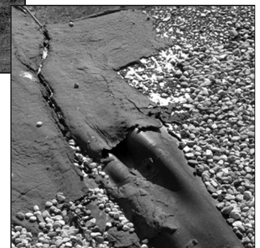
Photo 2 – Small, multipatch, split at re-entrant corner of EJ with failure to carry through.
