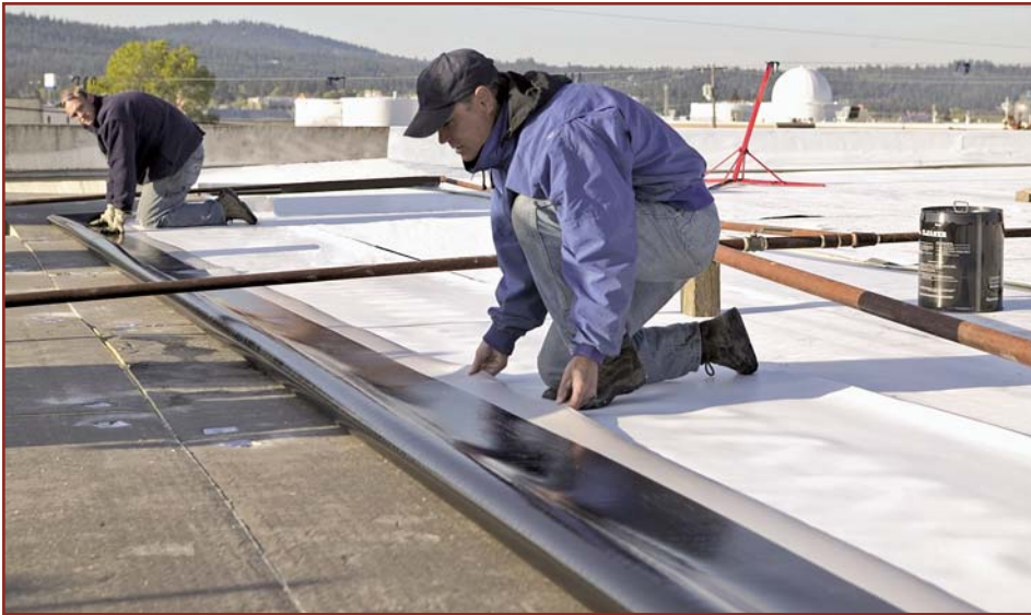
Photo 3 — Self-adhering TPO membranes provide easy installation, high performance, low VOCs, low odor, high reflectivity, and compliance with most environmental regulatory requirements.
