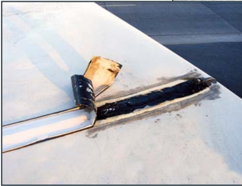
Figure 5 — Adhesive failure
