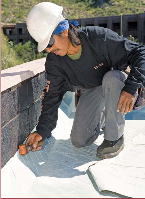
Photo 4 — Self-adhered base flashing for use under a heat-welded membrane.
