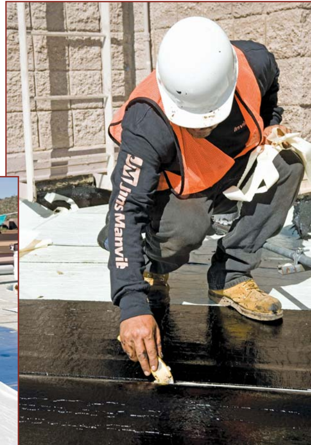
Photo 3 — Self-adhered membranes can easily be used in tight spaces.
