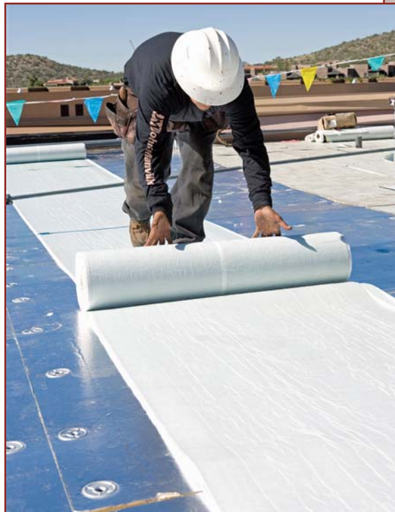
Photo 2 — Self-adhered membranes can be installed quickly to keep a building dry.
