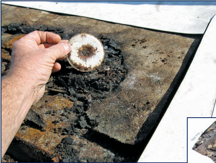
Photo 3 — The severely compromised locations are small but numerous and randomly dispersed. The roof area encompassed between 5% to no more than 10% of the deck area. The two buildings addressed were only six and eight years old. The deterioration is stunning and created a very real safety issue. We suspect deck failure will accelerate exponentially.
