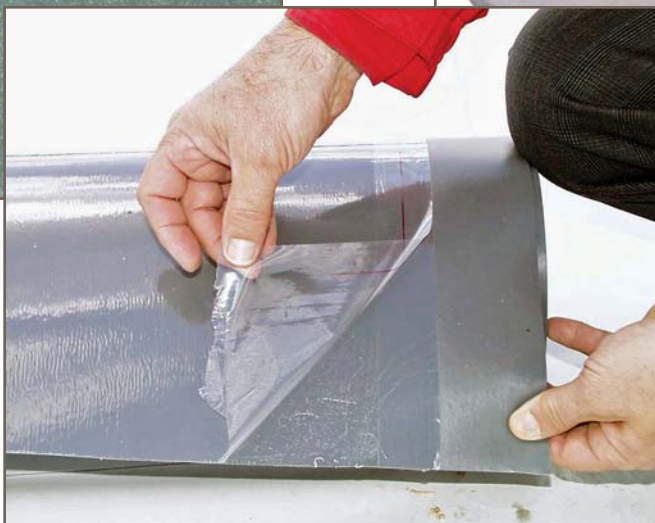
Photo 3 — Removal of backing from membrane
