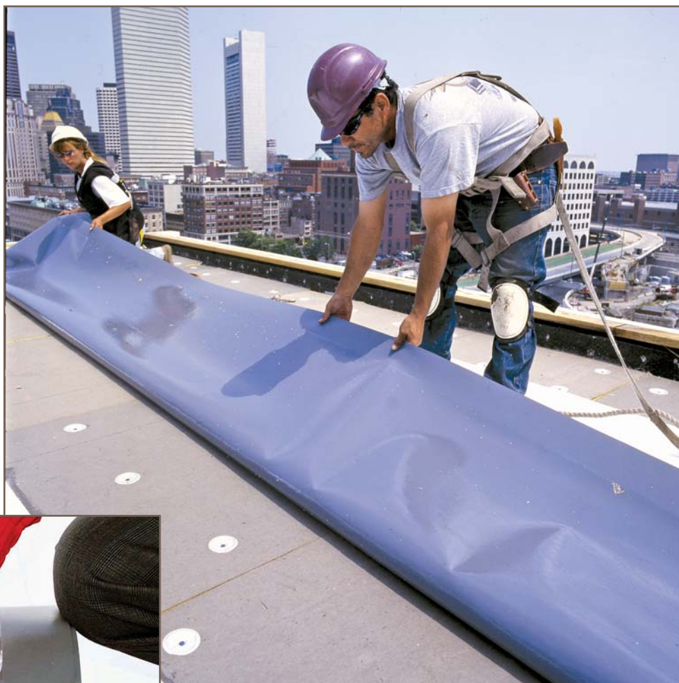
Photo 4 — Folding down membrane
