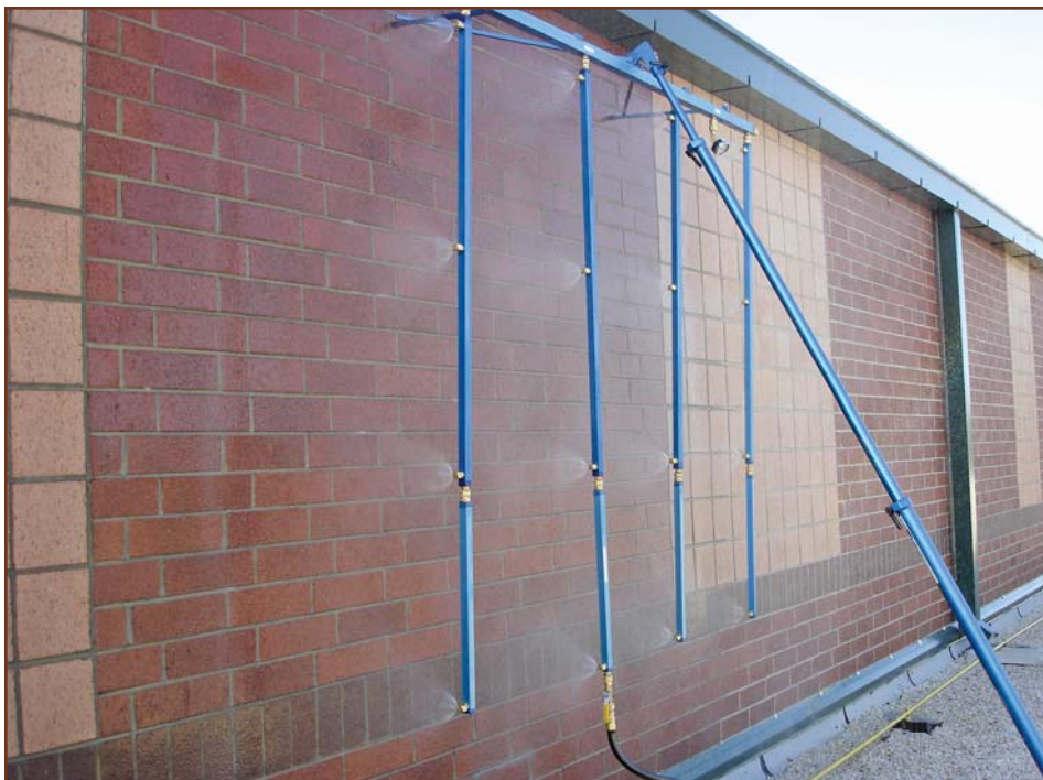
Figure 5 – Sheeting water created by water test.
