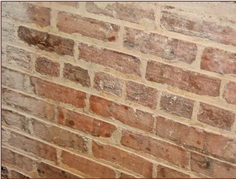
Figure 7B – Tooled flush joint, old construction.
