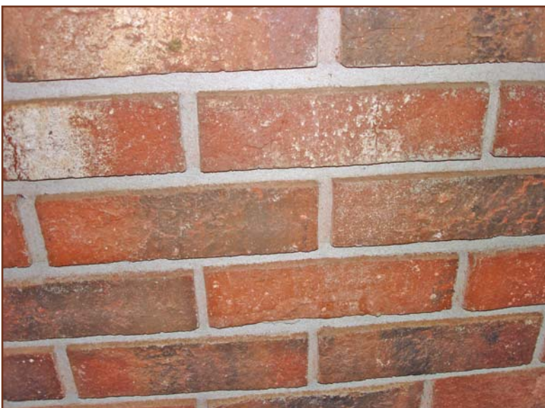
Figure 7C – Tooled raked joint.
