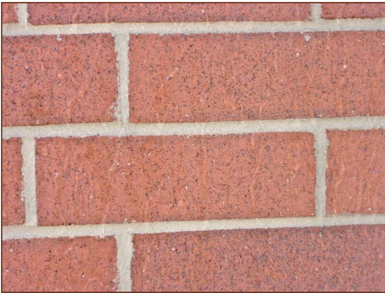
Figure 7A –Tooled concave joint.
