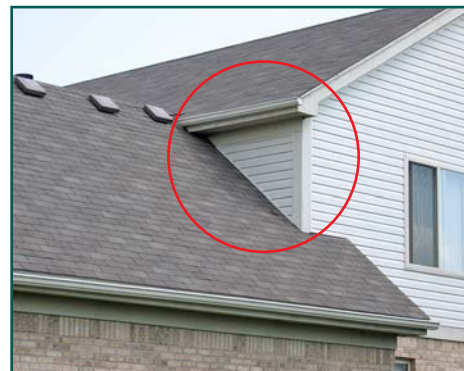
Photo 3 - Ridge intersecting eaves.
