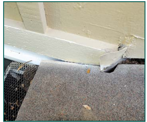
Photos 9 and 10 – Poorly fabricated kickout flashings will lead to water damage.
