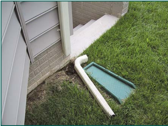
Photo 34 – Disconnected downspout.
