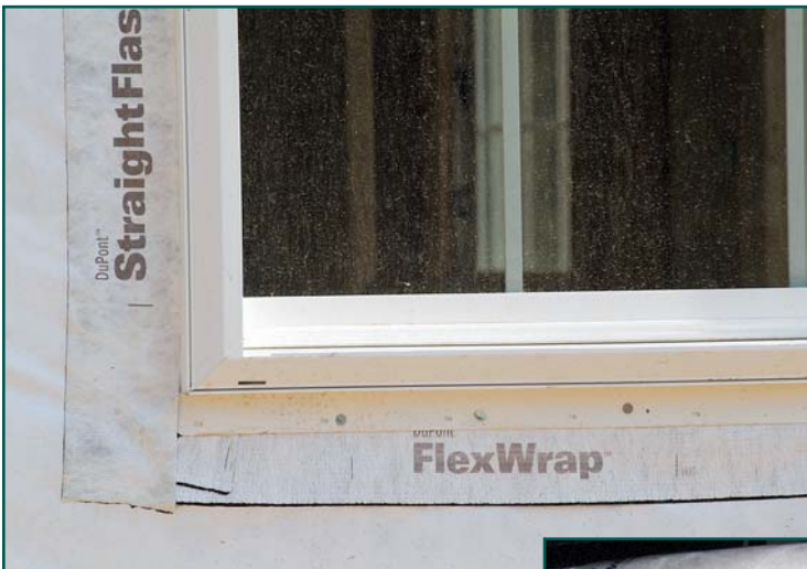
Photo 28 — Proper window flashing at sill. The sill flashing was installed before the window.
