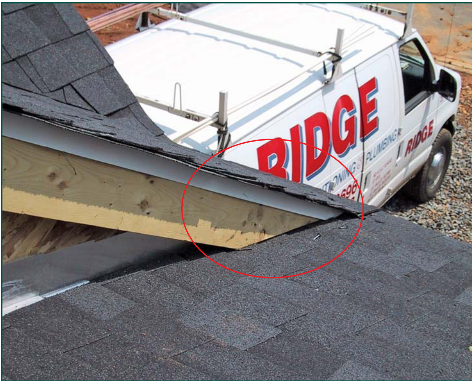
Photo 4 – Intersecting roof plane.
