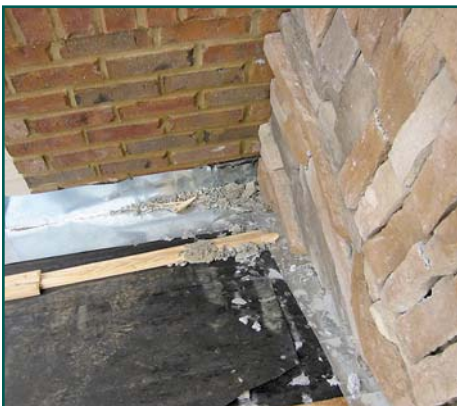
Photo 12 – Metal flashing reverse shingled over brick.
