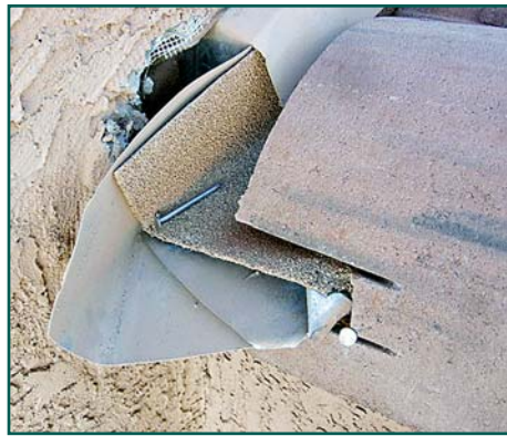
Photos 9 and 10 – Poorly fabricated kickout flashings will lead to water damage.
