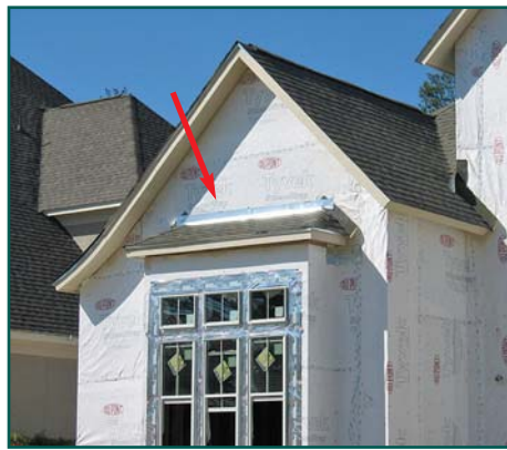
Photos 13 and 14 – Reverse-shingled weather barriers.
