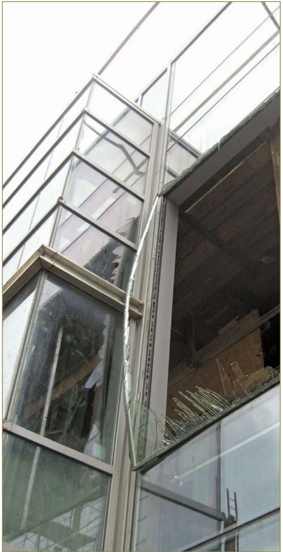
Photo 11 - Curtain wall after 150% design load test.
