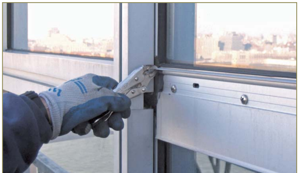
Photo 8 - Fixing pressure bar with pliers.
