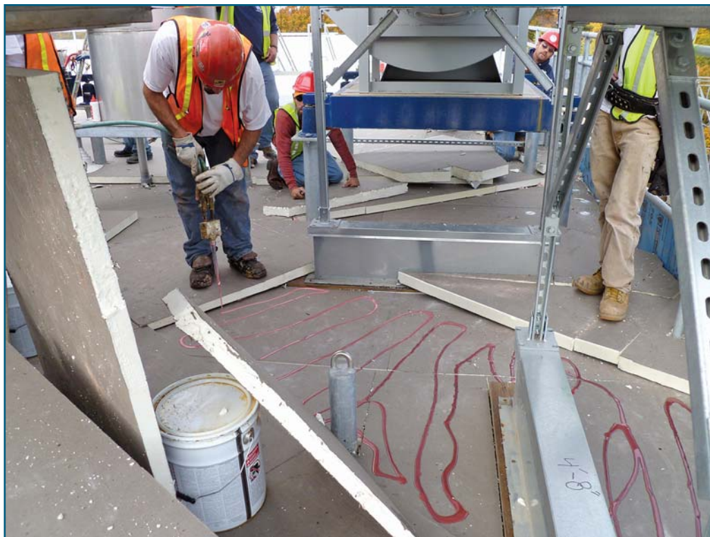
Figure 6 – Carts are ideally suited for larger projects where the roof is more open. Some carts have hoses as long as 30 ft, increasing mobility and production so that moving around the roof and providing coverage around penetrations do not pose problems.
