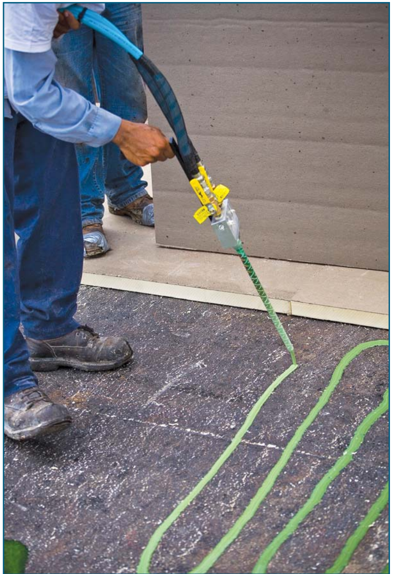
Figure 1 – Several industries preclude the use of mechanical fasteners that penetrate the roof deck. In addition, some owners and designers have gravitated toward environmentally sensitive “green” adhesive materials available on the market.
