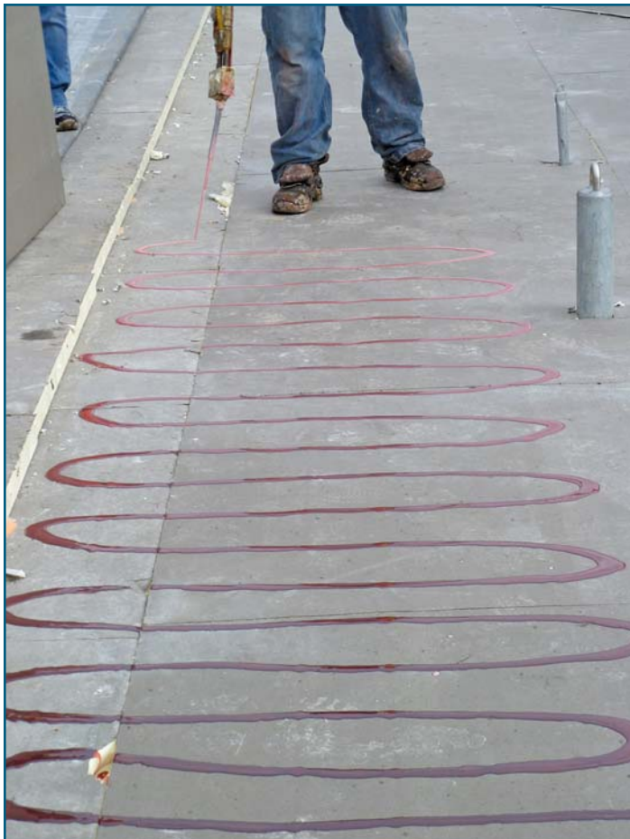
Figure 2 – Two-component, urethane-based adhesives were developed in the mid 1990s as an alternative to single-component urethane. These adhesives do not rely on ambient temperature or humidity for curing and thus provide a more predictable cure time and are typically installed in beads with a maximum spacing of 12 inches on center.
