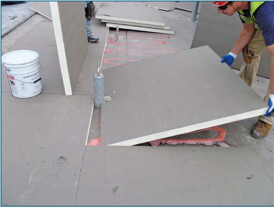
Figure 7 – Today’s two-component insulation adhesives are designed for use on virtually every common roof deck – steel, wood, concrete, gypsum, lightweight concrete, cementitious wood fiber, smooth BUR, smooth and granular modified bitumen, asphaltic vapor barriers, and fleece-backed vapor barriers. In addition, many can be used to adhere layers of insulation together.
