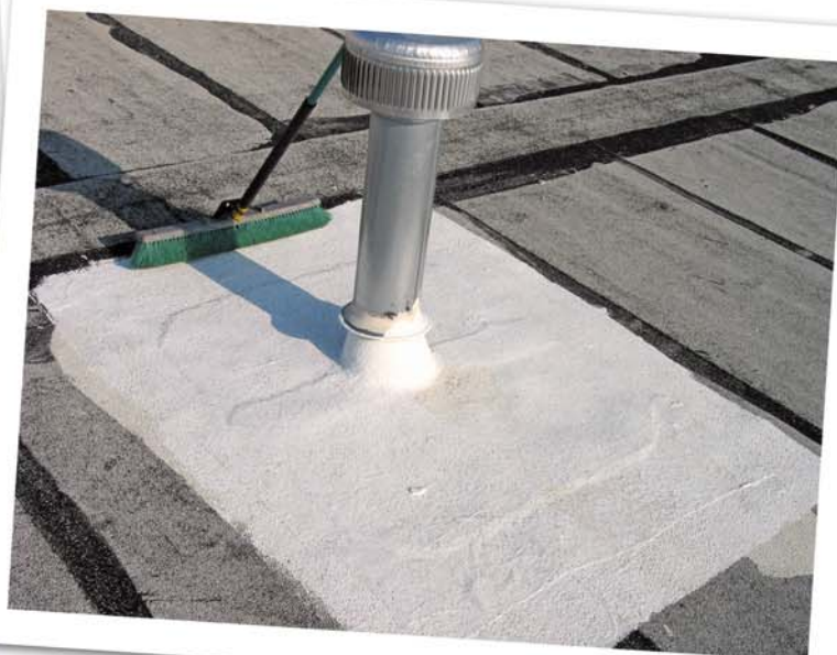
Detail of proper penetration repair using polyester scrim and coating.
