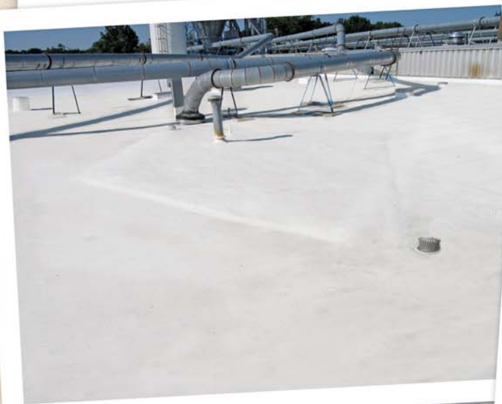
Valley line after resloping with SPF and coating.
