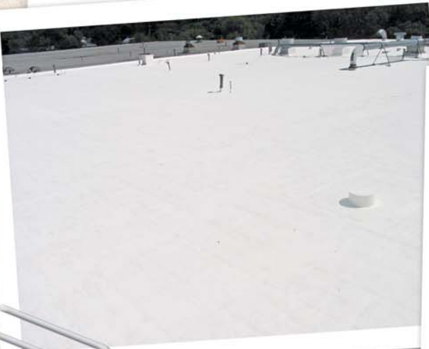
Field of roof of finished project.
