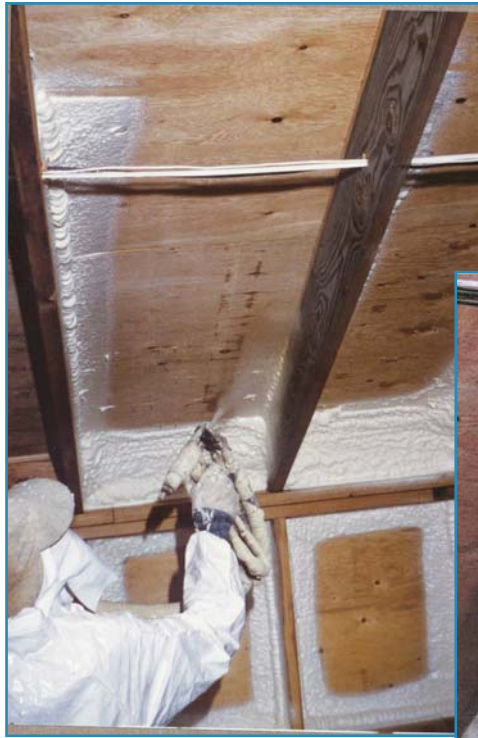
Photos 5 and 6 – Closed-cell foam should be installed in a “picture frame” technique to ensure uniform installation and to enhance adhesion to the studs.
