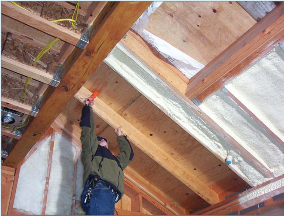
Photo 7 – Measure moisture content of the substrate before installing the foam. Wood substrates such as plywood and OSB should contain no more than 18% moisture as measured by a Delmhorst Moisture Probe (or equivalent measuring tool).
