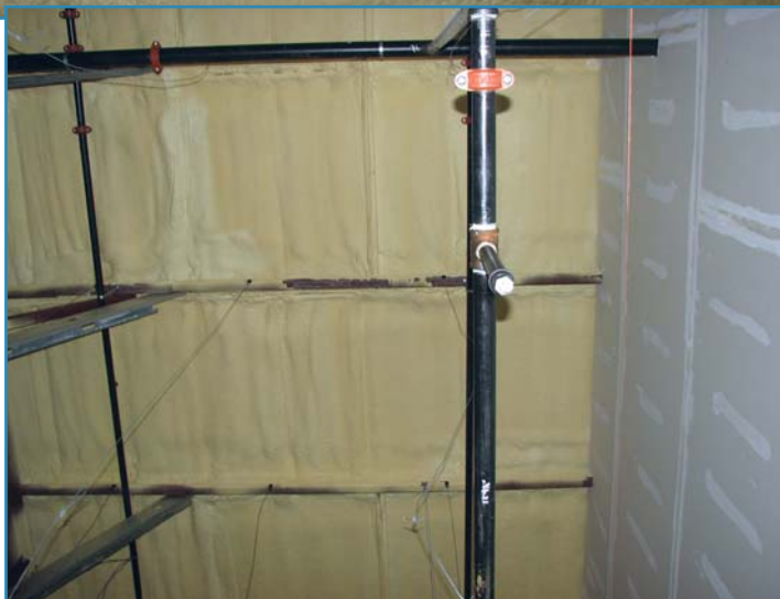
Photos 3 and 4 – Here, ccSPF is installed on the interior of a metal building without wall studs. This type of application has an added benefit of reducing thermal bridging through the metal beams and columns.
