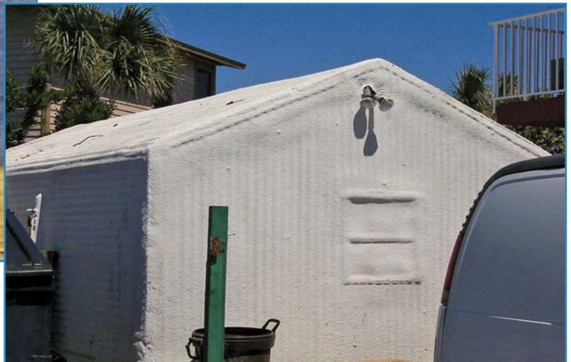
Photos 8 and 9 – ccSPF provides a water-resistant air barrier to the exterior of buildings, reduces thermal bridging, and can enhance the resistance of the structure to high winds and wind-driven debris.
