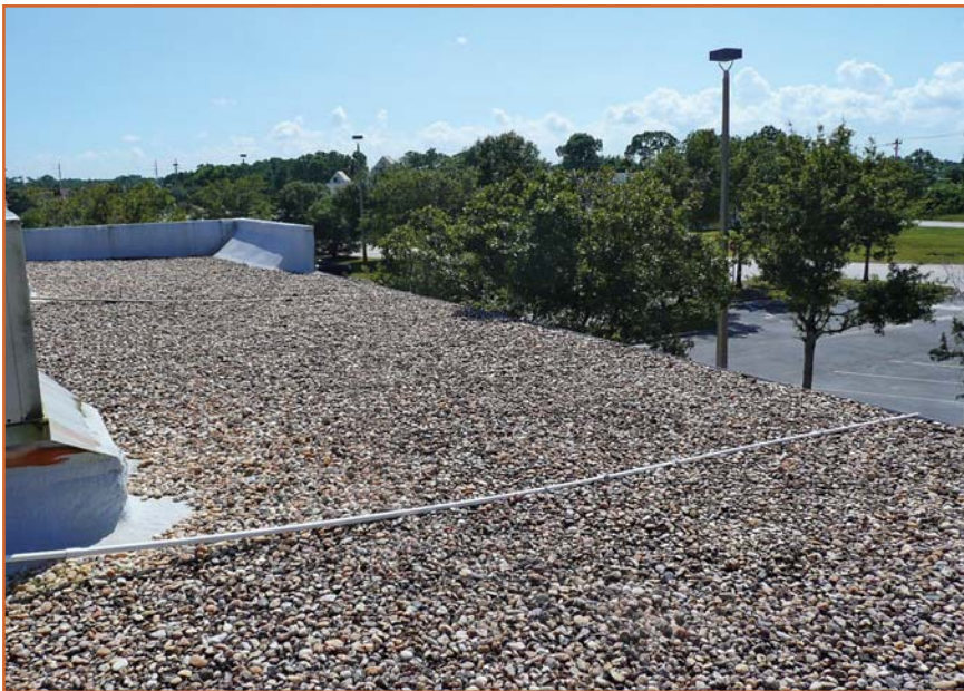
Figure 4 – Roof No. 19 with 1.5-in aggregate and a wrap-around parapet.
