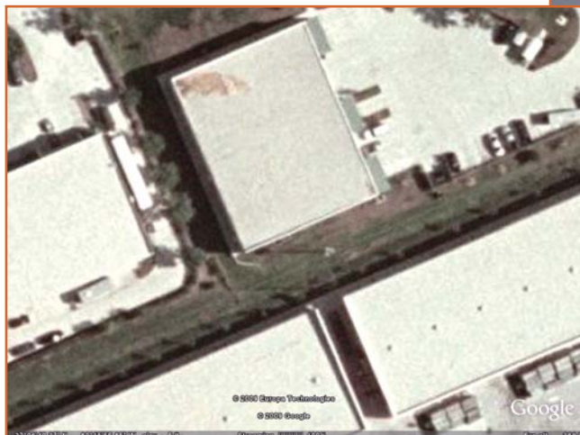
Figure 7 – Typical scour pattern (Roof No. 2). Photo courtesy Google Earth.
