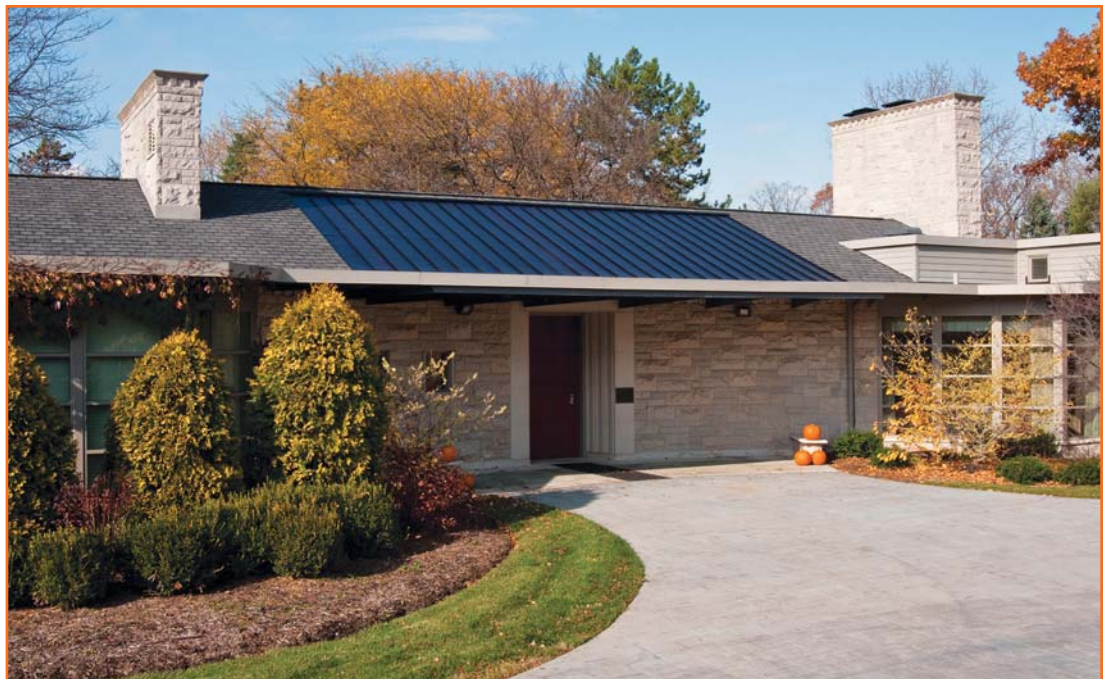
Photo 1 – A California home with an EnerGen™ PV solar power roofing system from CertainTeed. The EnerGen™ system features integrated UNI-SOLAR® thin-film laminates that integrate with traditional asphalt roofing shingles. Photo by C. Scott Widdes.
