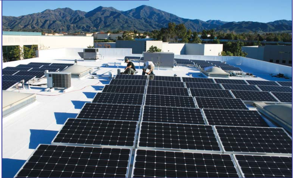
Photo 3 – Energy-efficient cool roofing systems can significantly reduce roof temperatures during the summer, improving the performance of the photovoltaic system. Photo courtesy of Coat’N’Cool.
