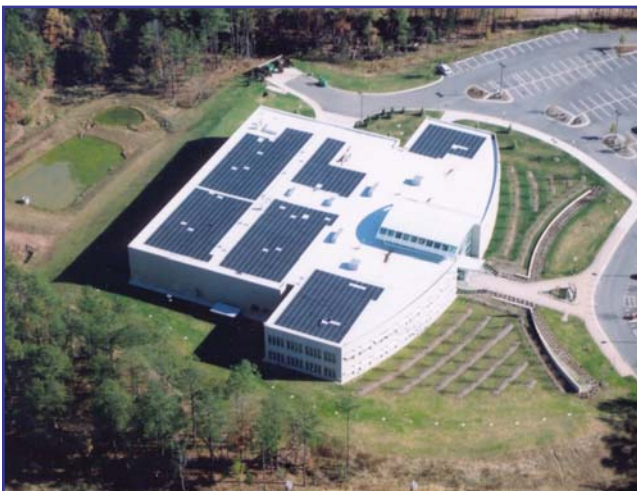
Photo 4 – One of the more prominent buildings that combines a cool roof with solar panels is the EPA’s 101,000-sq-ft National Computer Center in RTP, near Raleigh, NC. Photo courtesy of the EPA.
