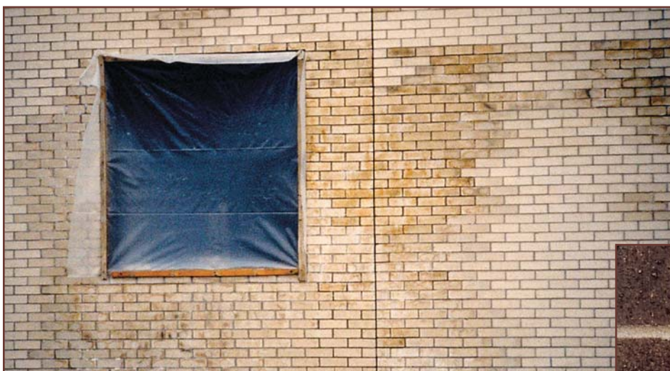
Figure 9 – Vanadium metallic stain leaves varied shades of yellow to light tan to light green splotches. (Courtesy of PROSOCO.)
