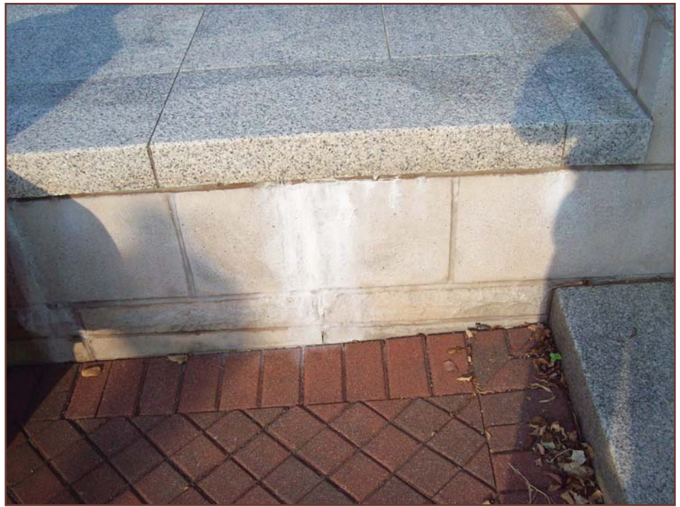
Figure 11 – A form of lime run beginning at the mortar joint and trailing down the face of the masonry.
