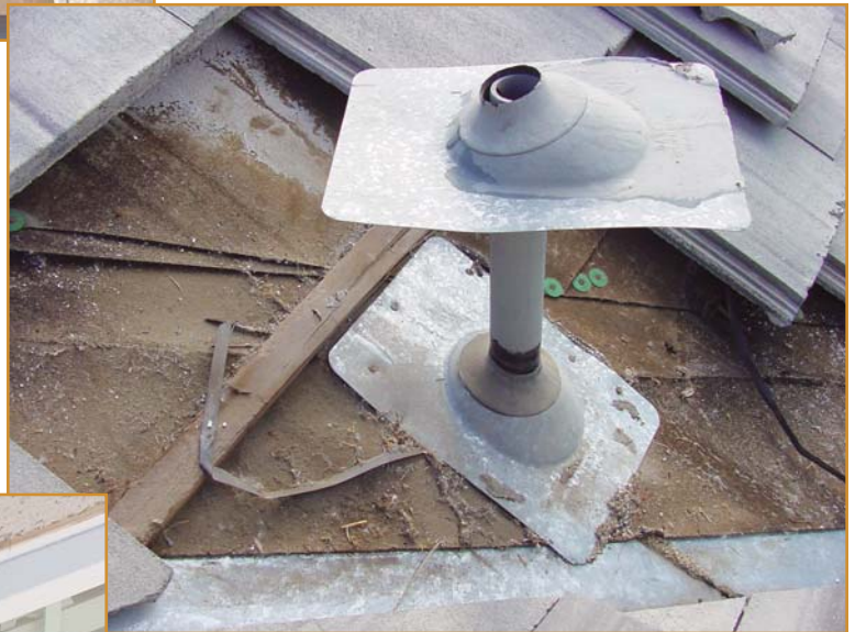
Photo 4 – The integration of penetrations through the roofing requires that the roofing subcontractor work with the plumbing subcontractor to ensure that the lower flashings are integrated in a shingle-lapped manner and sealed, and that the upper flashings are integrated with the tile and sealed. In this case, the penetration near the valley is a problematic detail that should not occur. Simply put, keep holes out of valley construction.
