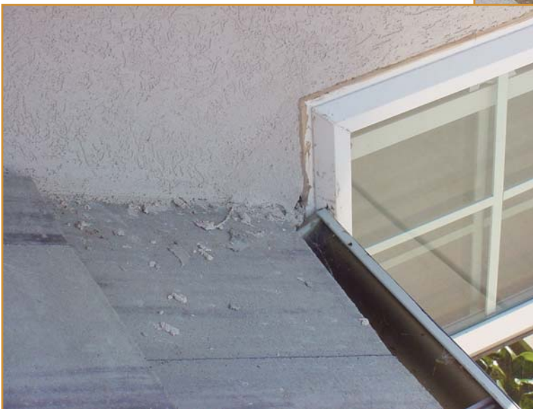
Photo 5 – The integration of the flashing from the roofing and the sidewall cladding is extremely important. The roofing subcontractor must ensure that the roofing felts, waterproofing, continuous flashing, and diverter flashing are all coordinated so they lap properly. A situation like the one in the photograph above should be brought to the attention of the designer of record. The window is damaged due to the location of the gutter, and because without flashings, water is directed into the jamb of the window. Contractors and subcontractors should not proceed with their work until such situations are fully resolved.
