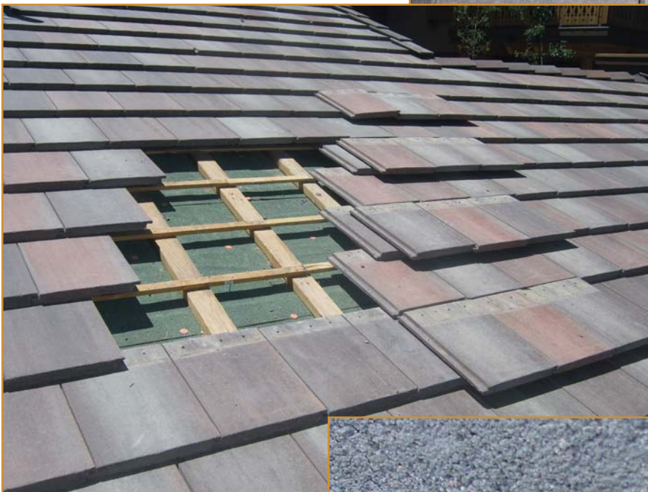
Photo 11 – The vertical battens must be nailed in order to transfer the wind load; after that, the horizontals must be nailed to the verticals, then the tiles to the horizontals. If not, there must be sufficient weight to resist wind uplift. Roof edges will have sufficiently increased uplift loads and will require additional fastening or clipping.
