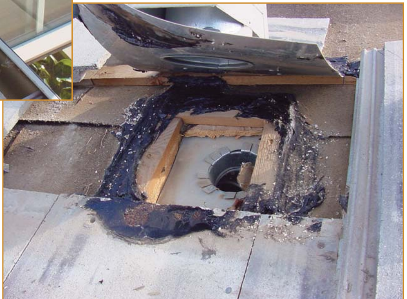
Photo 6 – The lapping of flashings and all moisture-management materials should ensure that water is directed down, out, and away from the roofing felts. In no case should mastic or sealant be relied upon to correct deficient construction.
