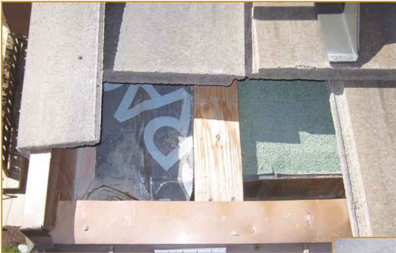
Photo 3 – The vertical batten prevents water in the channel from draining into the gutter below. The ice and water shield products must be properly integrated with the thermal envelope and the weather-resistive decking materials.
